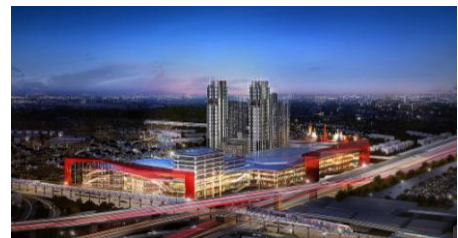
Bangkok Mall, Due for completion in 2017
